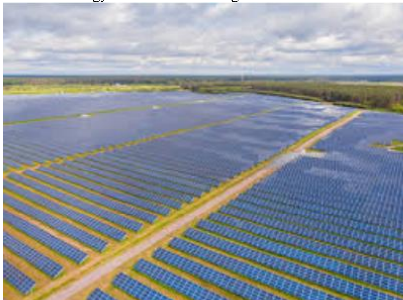
Figure 2. Large-Scale Utility-Scale Solar Energy Project
