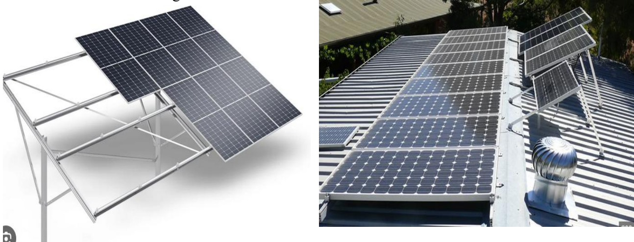
Figure 1: Mounting the solar panels (ground and Roof-mounted
