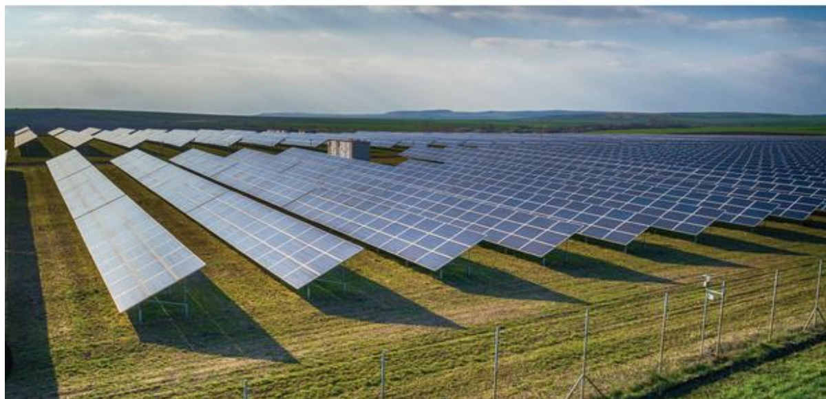
Figure 12. Utility-Scale Photovoltaic Systems Source: energy.mit.edu/news/solar-photovoltaics-the-benefits-outweigh-the-costs/
